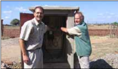
Andy & Chris officially switching on the power
