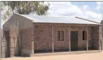
Community Housing being constructed
