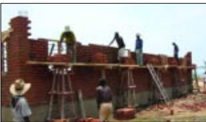
New duplex nurse's residence currently under construction.
